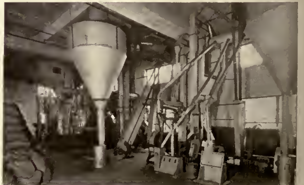
VIEW IN COFFEE-ROASTING ROOM ON SIXTH FLOOR
